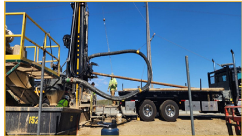
Drill Rig at IEUA's AR-MW-03 location
