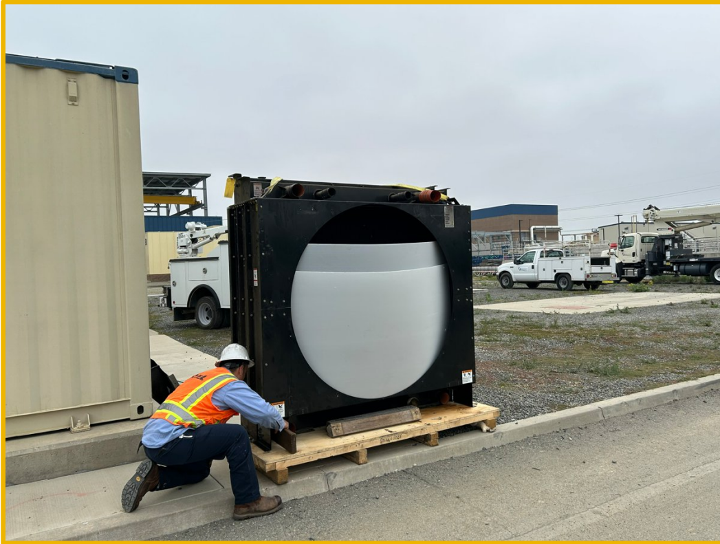
Old Unit Removed
