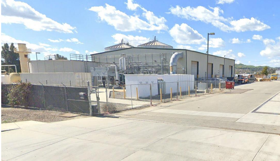
Typical Site View Mountain Ave Pump Station
