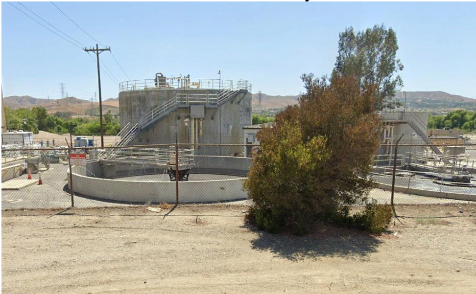
View of RP#2 Facility
