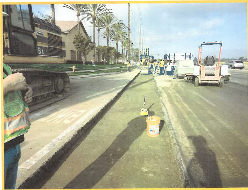
Base Paving After Pipe Installation
