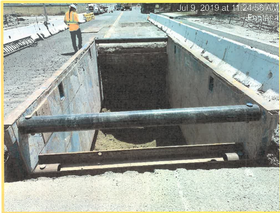
Bore Pit on Napa Street
