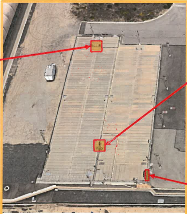
Chlorine Contact Basin 1B and 2
