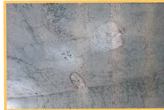
Sample Roof Sand Blasted Area
