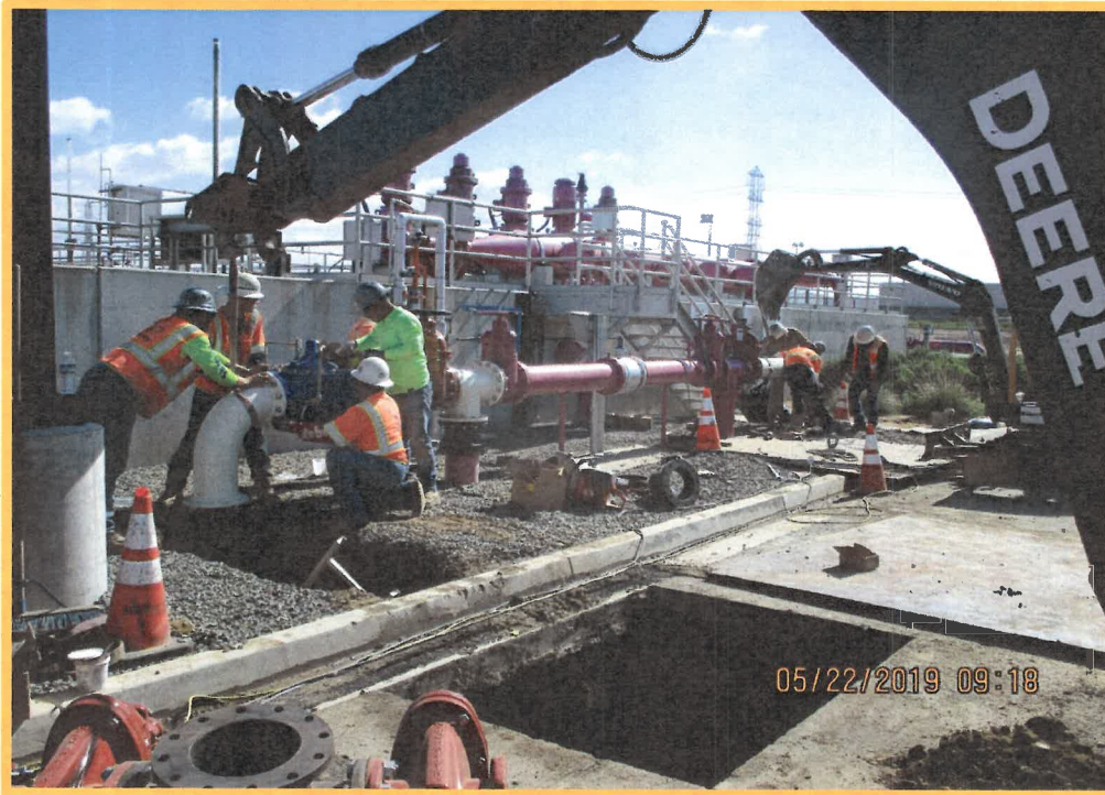
Piping Upgrade in Progress
