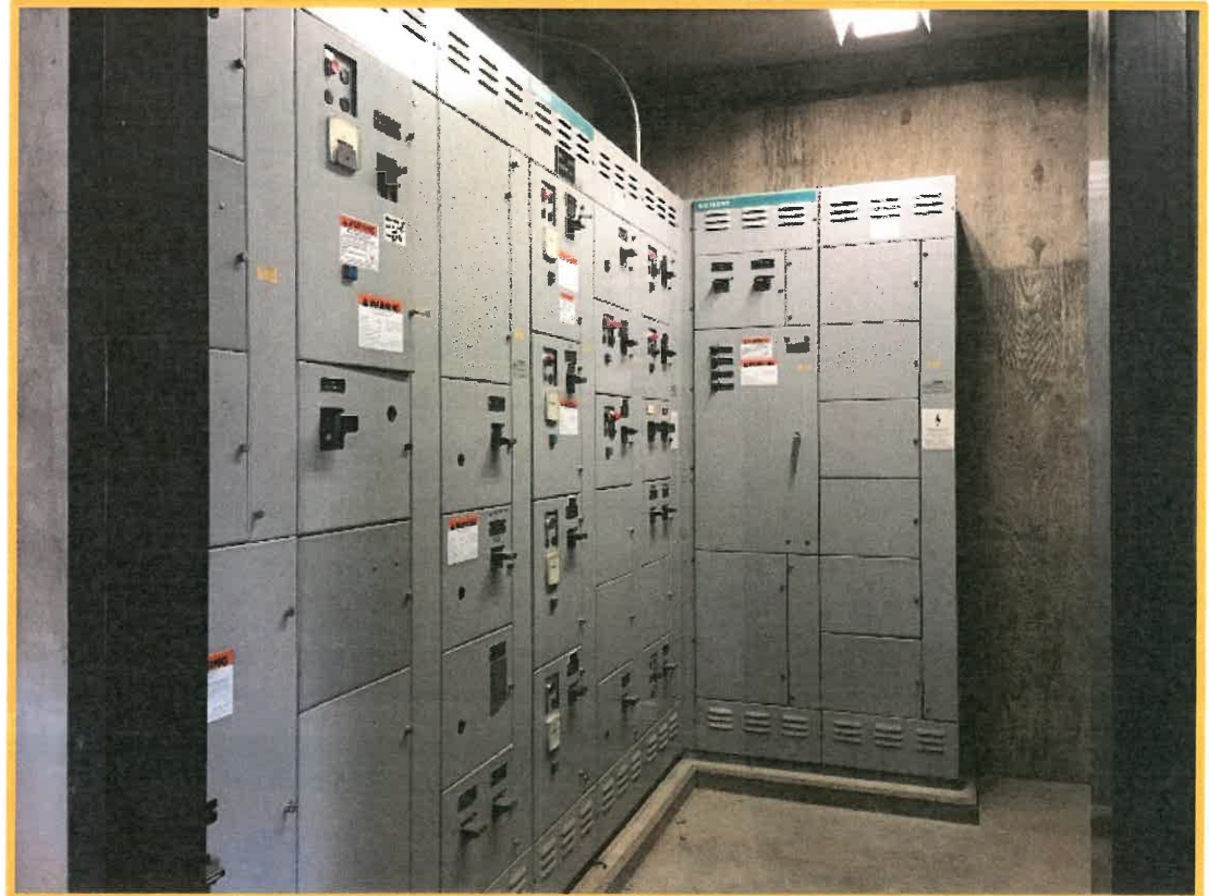
Building E - Old Motor Control Center Equipment
