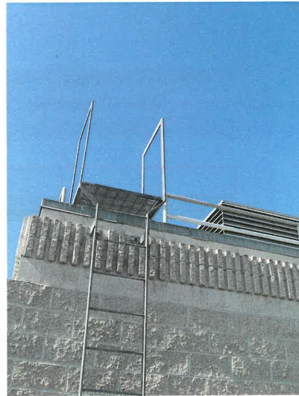
Fixed Ladder on PRB Building
