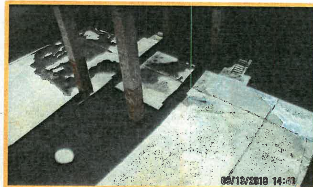
After Dewatering 09/13/18 2:40 PM
