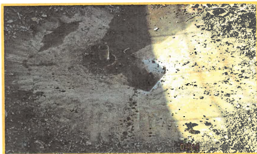
After Dewatering 09/19/18 8:43 AM
