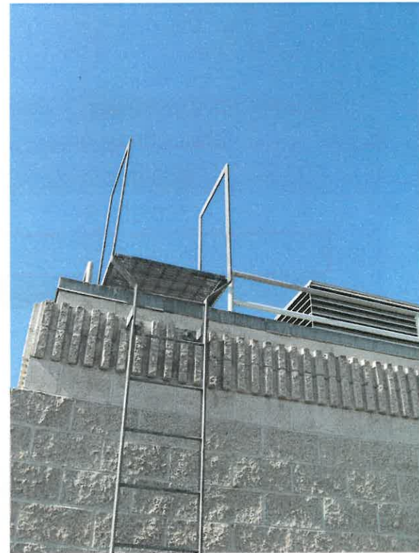
Fixed Ladder on PRB Building
