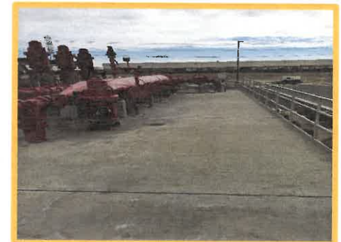
Location of New Wetwell Access Hatch
