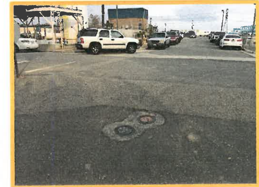
Sample Location - Non-Functional Buried Isolation Valves
