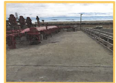
Location of New Wetwell Access Hatch
