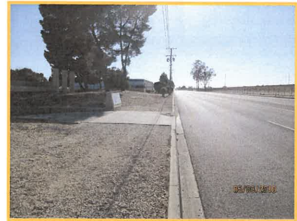
Philadelphia Lift Station
