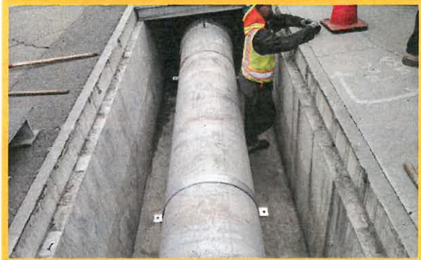
Straps Installed to Limit Duct's Displacement
