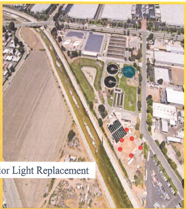
CCWRF Aerial Photograph
