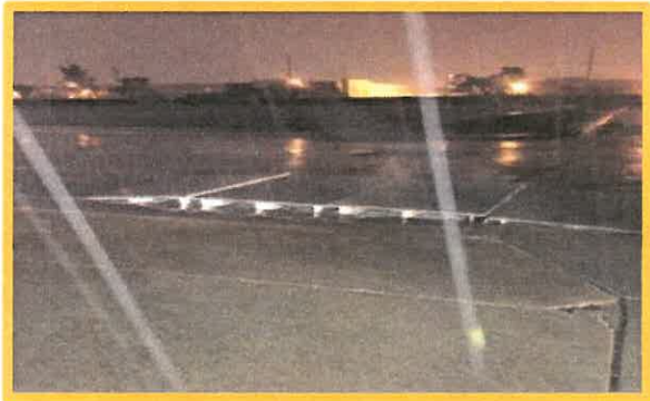
Vault Covers Floated During Winter 2017 Rain Event
