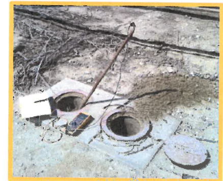
Corrosion Potential Measurement
