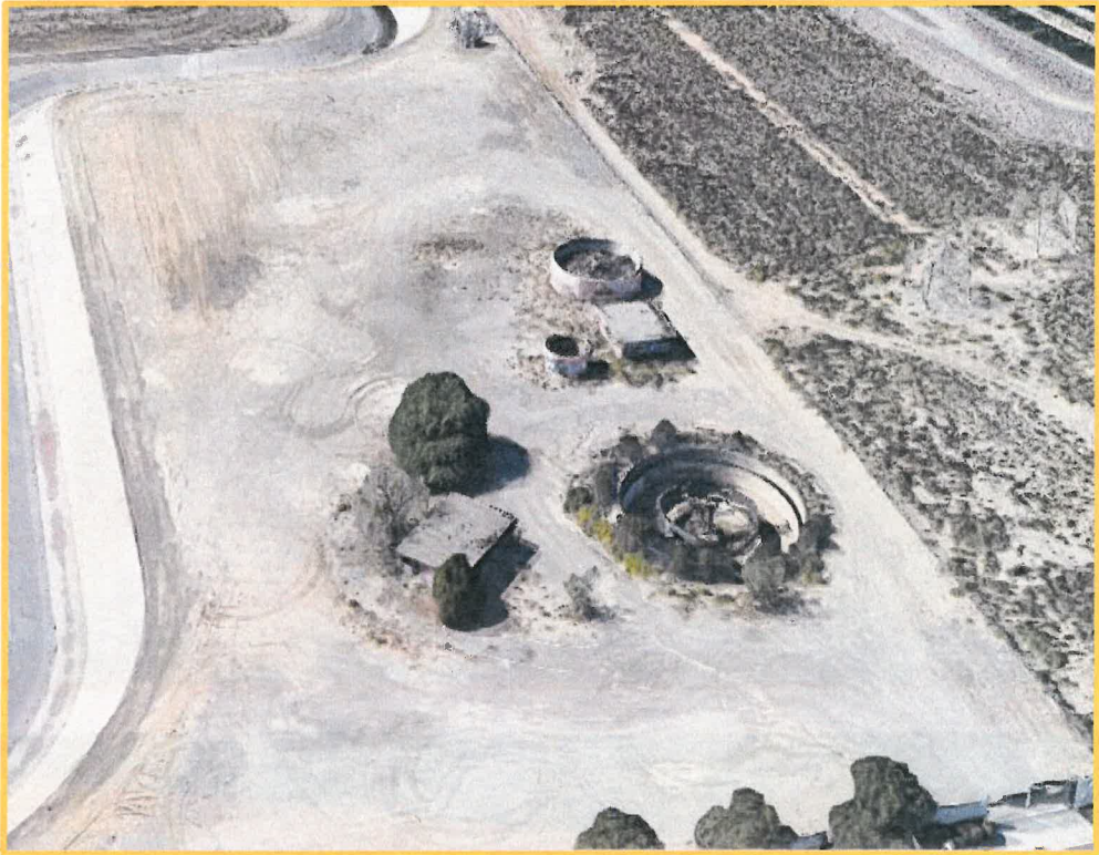
Aerial of Remaining Abandoned Structures
