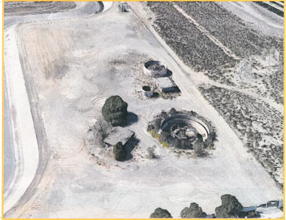
Aerial of Remaining Abandoned Structures
