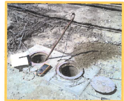
Corrosion Potential Measurement
