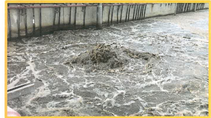
Aeration Basin Surface Boil
