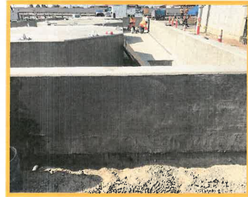
New Chemical Area with Tank Pad
