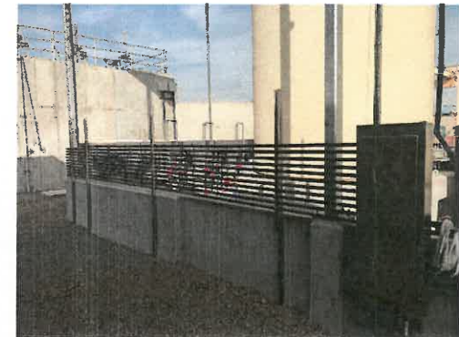
New Electrical Conduits to the Chemical Pumps
