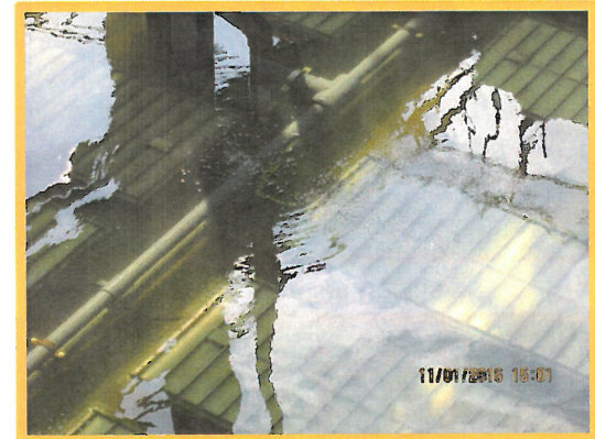
Air header leak during panel testing
