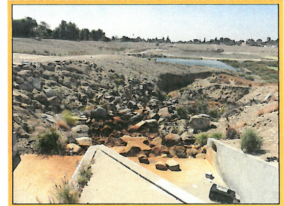
Existing Pipeline Discharge
