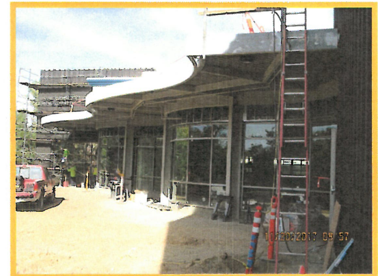
Lab Building Entrance Canopy
