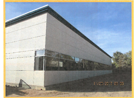
Lab Building North Side
