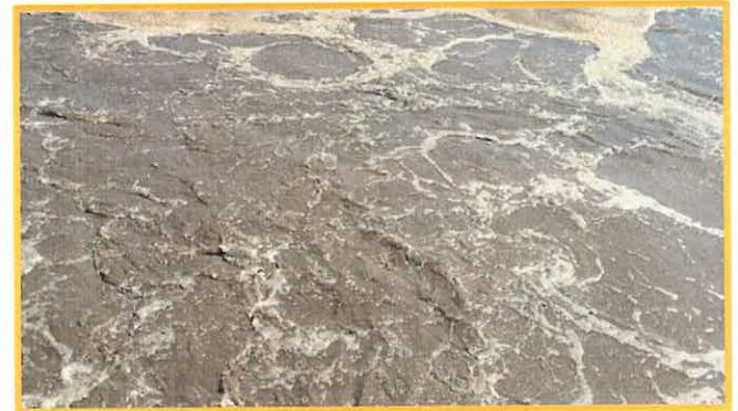
Boiling mixed liquor suspended solids prior to work
