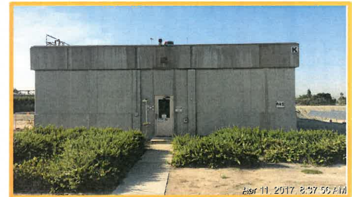
RAS Pump Station Building
