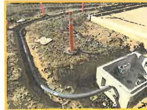
New Chemical Piping and Pull Box
