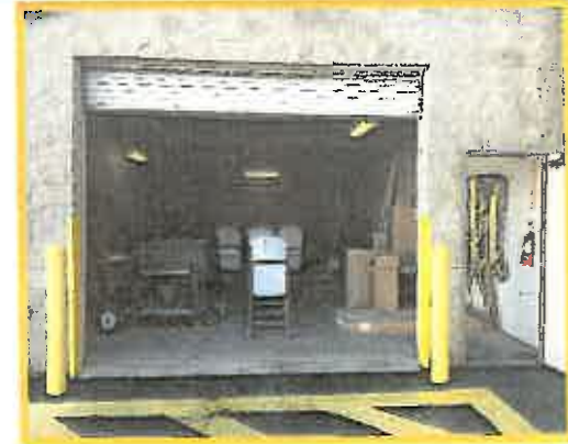
Existing Paint Room
