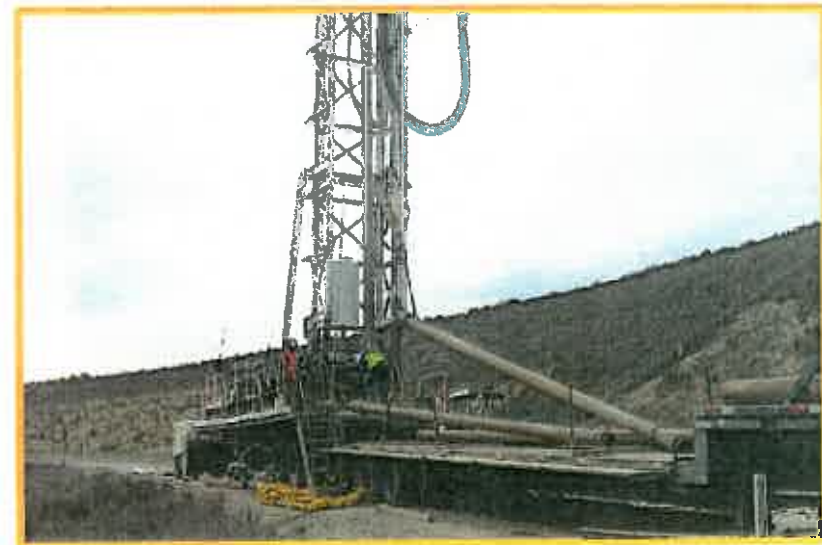
Past Construction of a Monitoring Well for San Sevaine Basin
