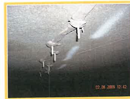
Digester Roof Repair (Internal)
