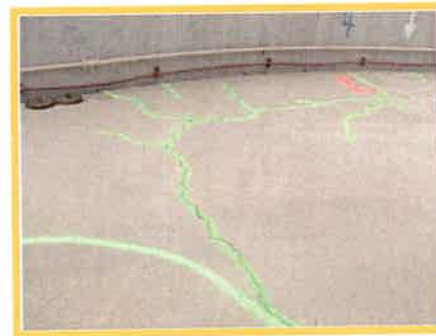
Digester Roof Repair (External)
