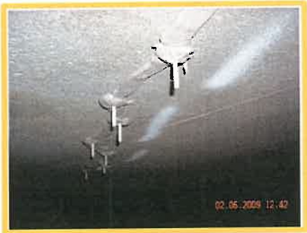
Digester Roof Repair (Internal)
