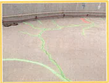
Digester Roof Repair (External)
