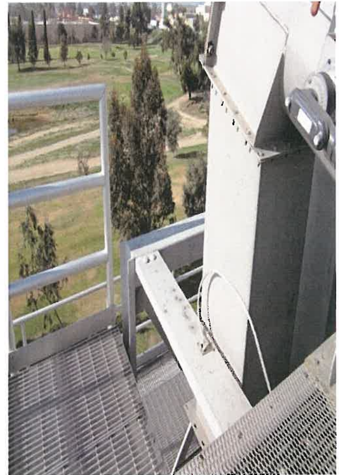
Location of Additional Railing
