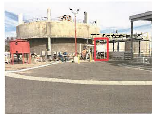
Acid Phase Digester Iron Sponge
