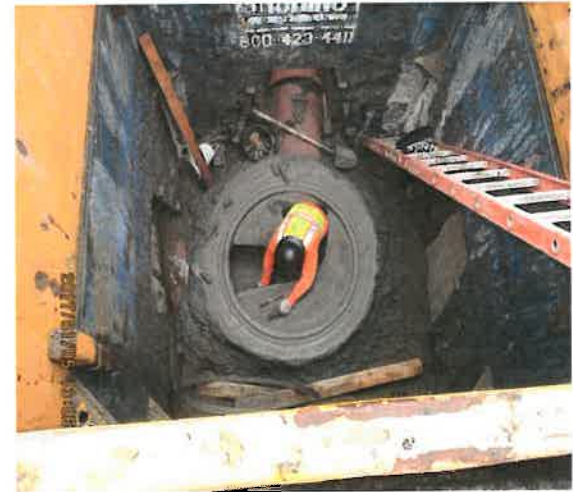
New 18-in Manhole Base
