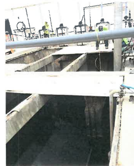
Corroded Concrete
