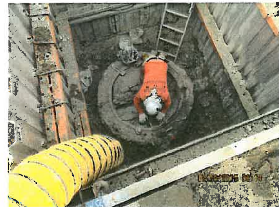
New Manhole Construction Over the Existing
