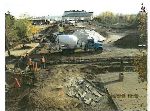
Trench Backfill and Compaction
