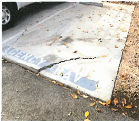
Typical Root Damage to Parking Slabs
