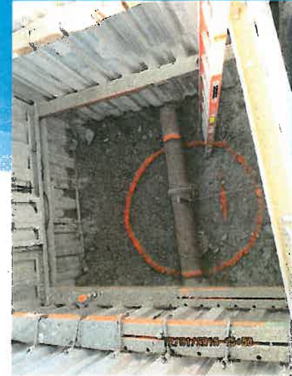
Connection Point for New 8-In Sewer Lateral
