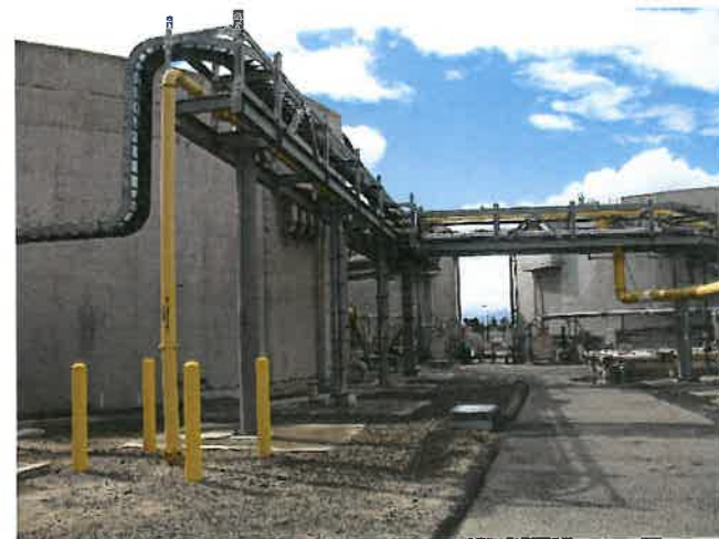
Partial Digester Area
