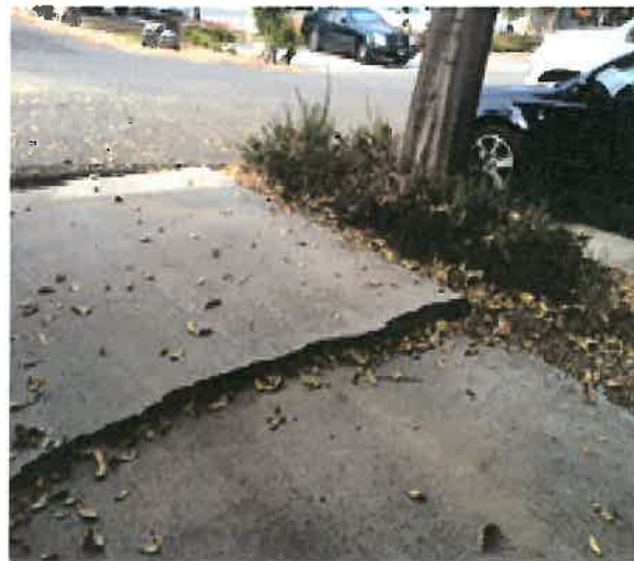
Typical Root Damage to Parking Slabs
