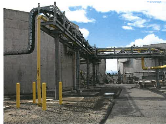
Partial Digester Area
