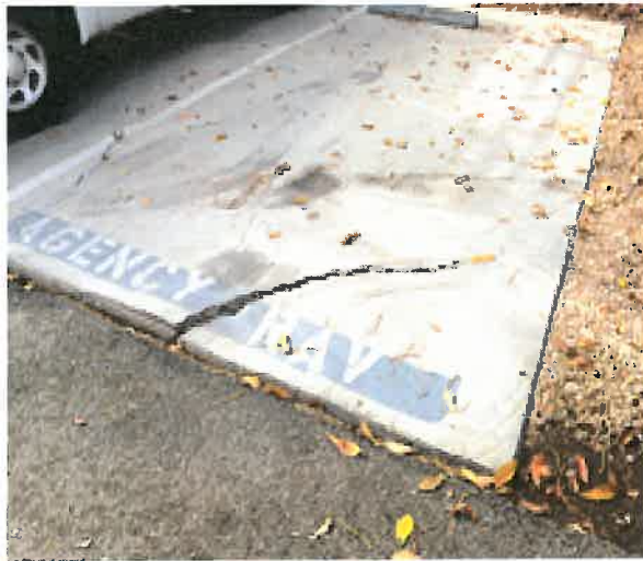
Typical Root Damage to Parking Slabs
