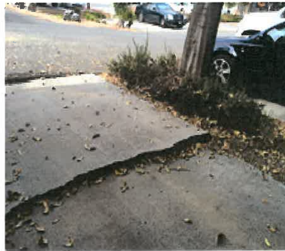
Typical Root Damage to Parking Slabs
