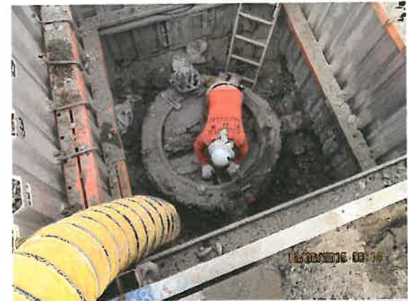
New Manhole Construction Over the Existing
