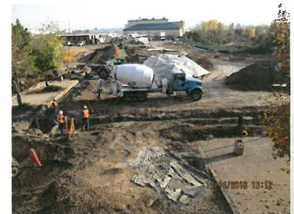
Trench Backfill and Compaction
