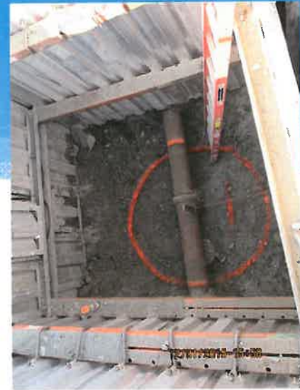
Connection Point for New 8-In Sewer Lateral
