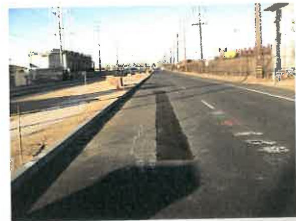
Backfill after Potholing
