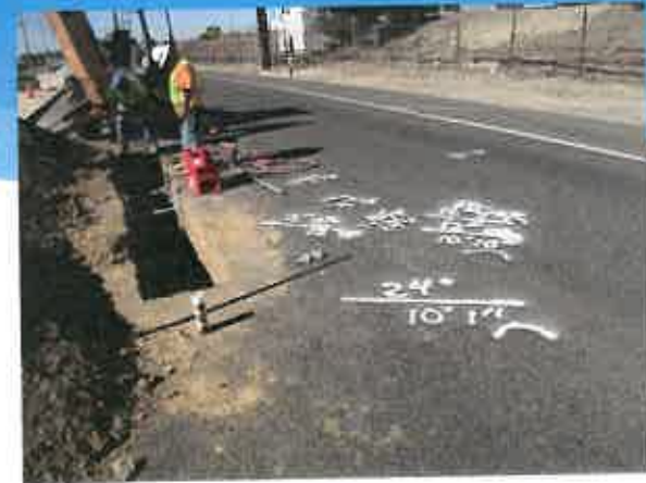
Potholing in San Bernardino Avenue
