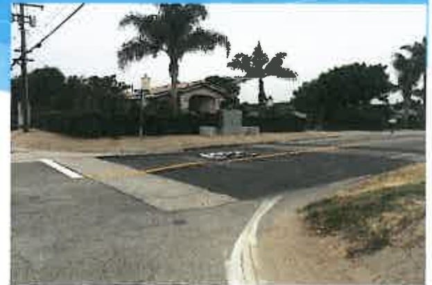
New Control Panel Installed & Street Paved
