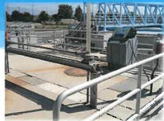
Primary Effluent Diversion Structure
