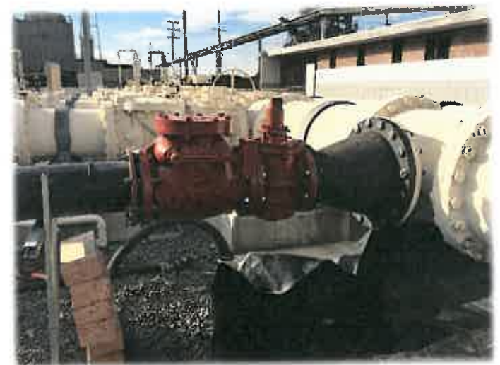
Temporary sewer bypass at SBLs
