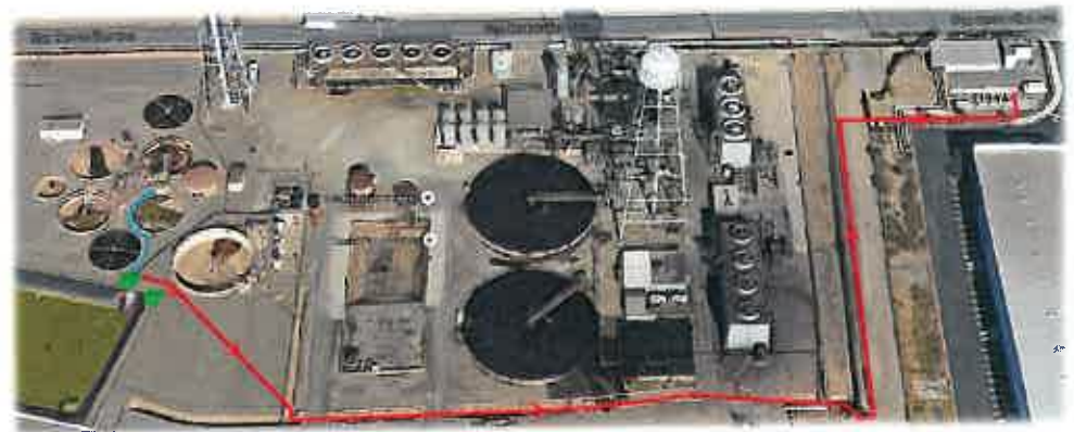
Temporary Bypass Sewer
