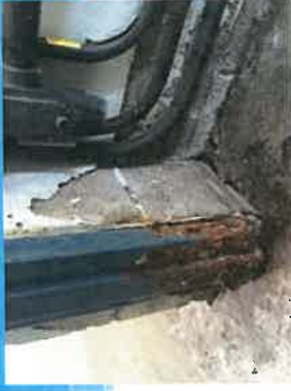
Corrosion Outside Containment Area
