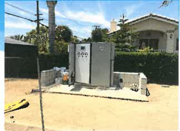
New VCP-100 Installed
