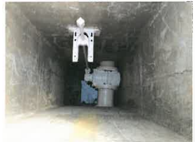
Top down view of newly installed 10" DAFT Valve
