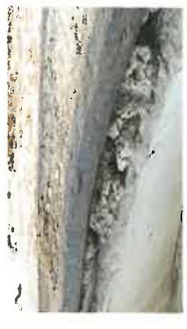
Deteriorated Grout
