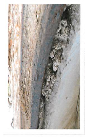
Deteriorated Grout
