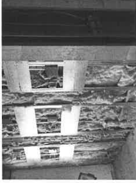
Control Room Wall Modifications
