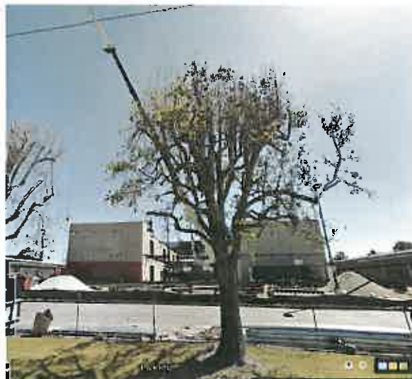
Example of schools construction: Digital image of construction in progress at Ontario High School obtained from "Google Maps – Street View", 2015
