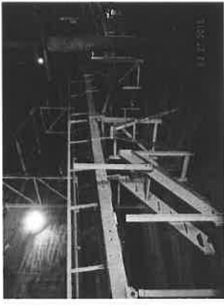
BC-18 After Mod's, Catwalk Installation Ongoing
