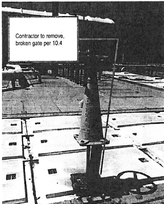
10.6 Grit Chamber and Primary Influent Diversion Channel Picture
