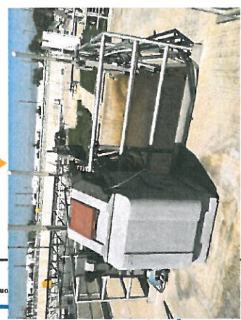
Secondary Clarifier Splitter Box
