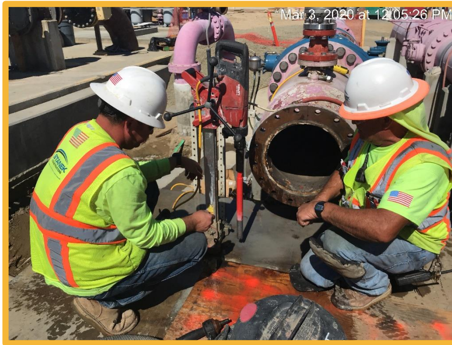
Drilling Anchors for New Pumps
