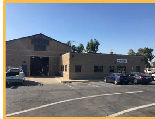
3 TP-1 Maintenance Building
