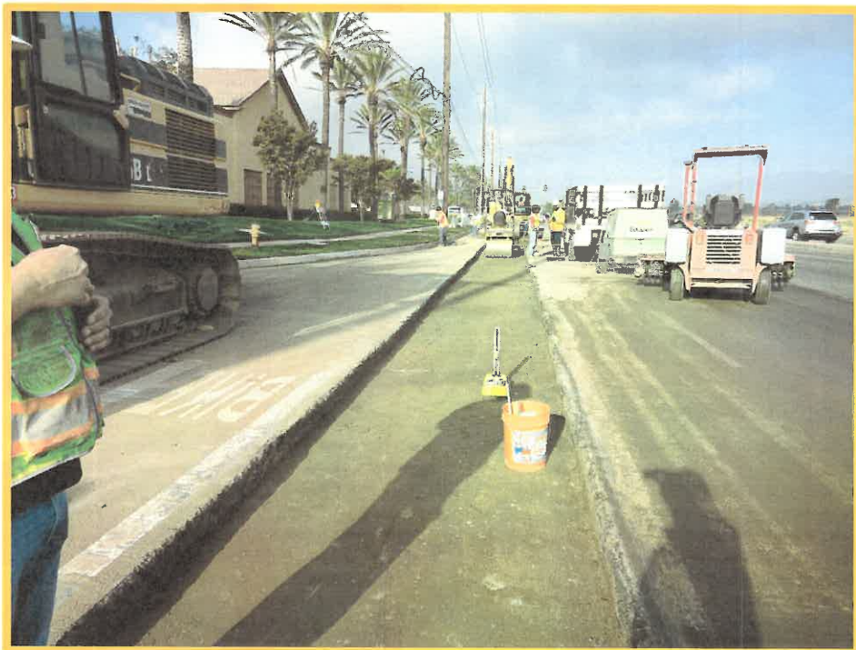
Base Paving After Pipe Installation
