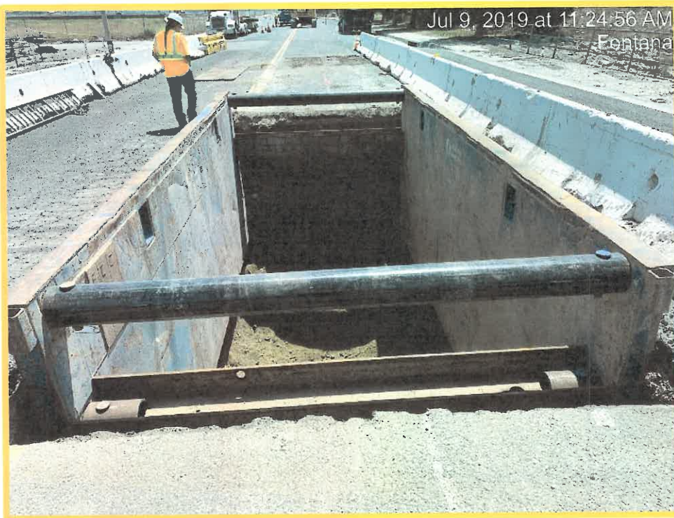
Bore Pit on Napa Street
