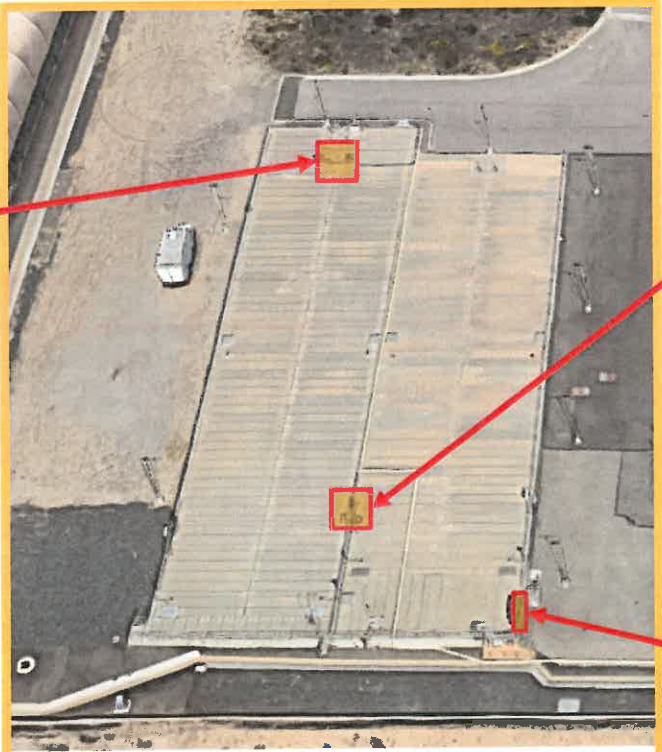
Chlorine Contact Basin 1B and 2
