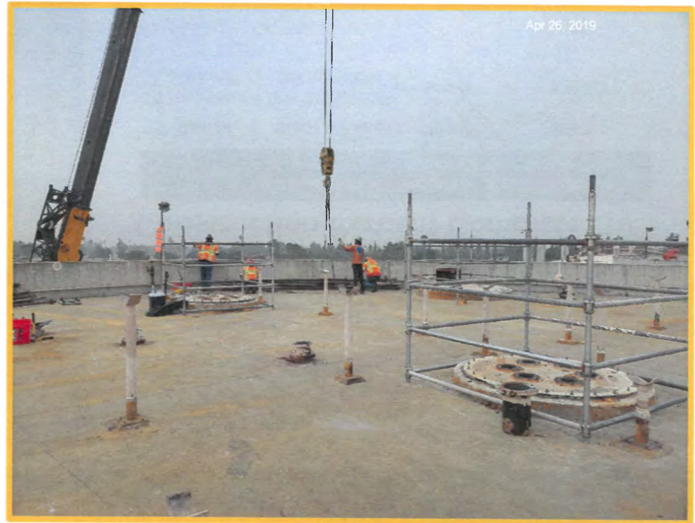
Digester 6 Gas Pipe Removal
