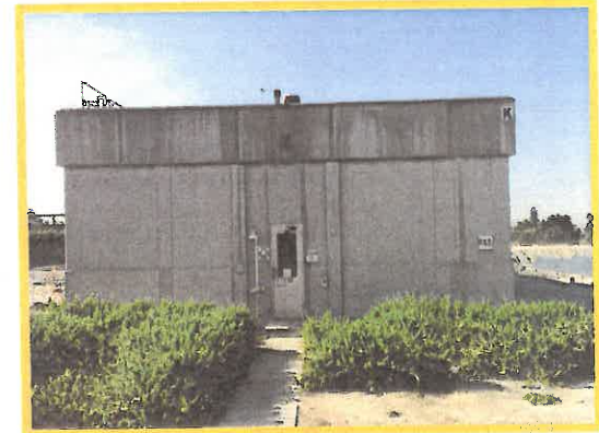
Building E Pump Station
