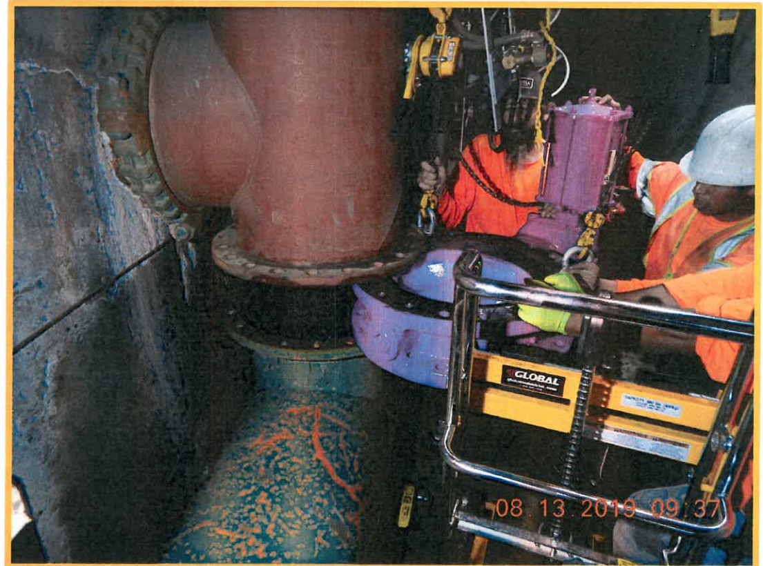
New 20-inch Filter Valve
