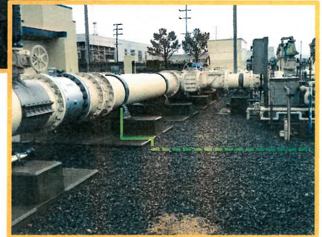
Proposed Drain Line Location
