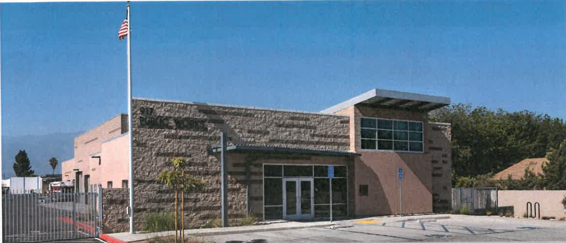
built- San Gabriel Municipal Yard
