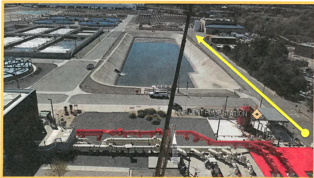
Influent Pump Station Overflow Pipeline Location
