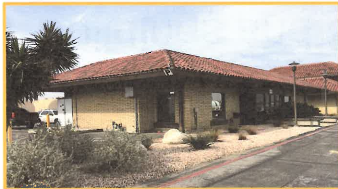
Westside of Cucamonga Creek Channel Admin/Lab Building letter "A"
