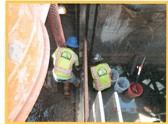
Installation of Isolation Bulkhead
