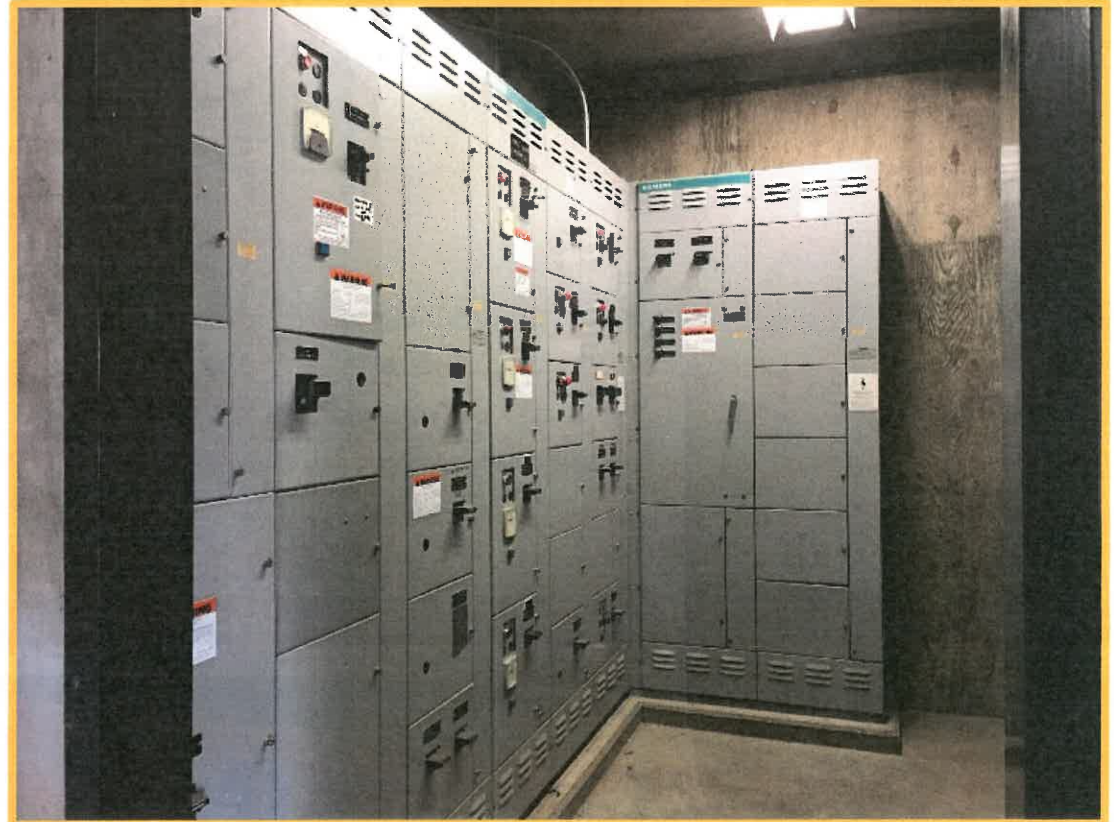
Building E - Old Motor Control Center Equipment
