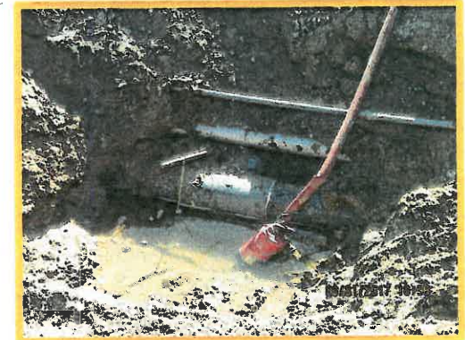
RW Pipe Rupture Repair Due to Surge
