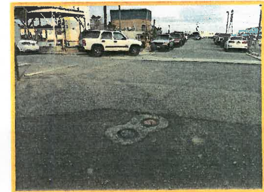
Sample Location - Non-Functional Buried Isolation Valves
