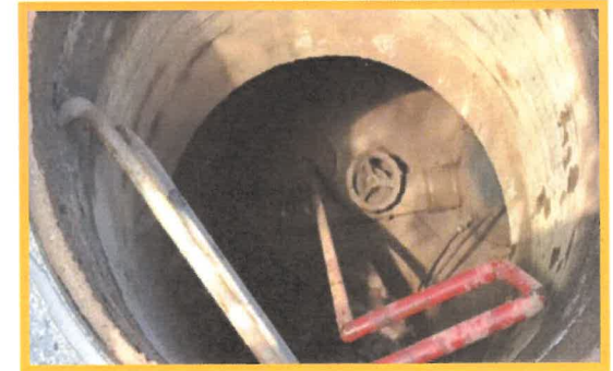
Existing Flow Meter Manhole
