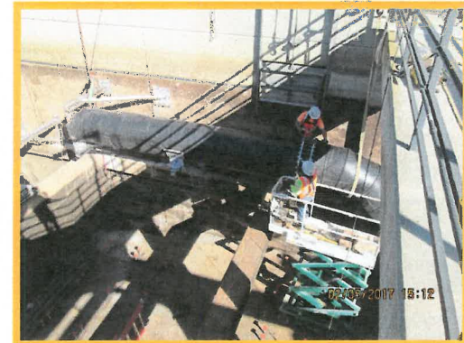
New 36" Dia. MLR Piping installed
