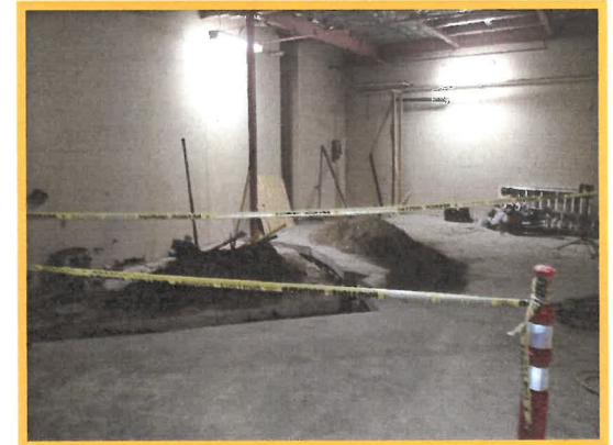
New Drain Pipe Trench
