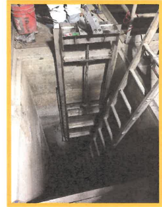
Setting New Gate in Place
