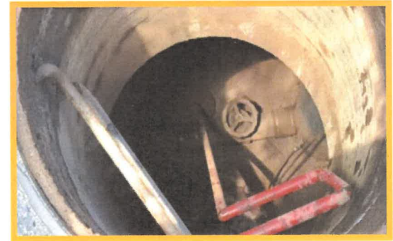
Existing Flow Meter Manhole
