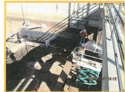
New 36" Dia. MLR Piping installed
