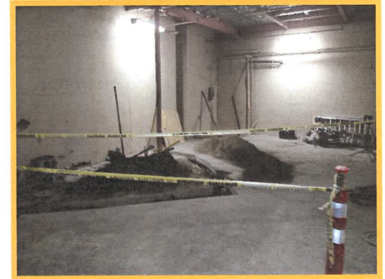
New Drain Pipe Trench
