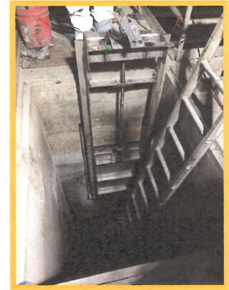
Setting New Gate in Place
