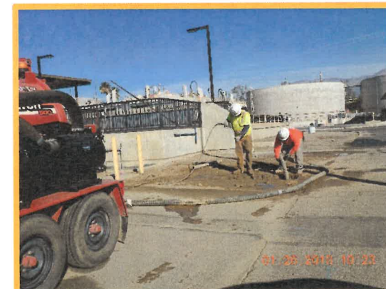
Potholing for Scum Piping
