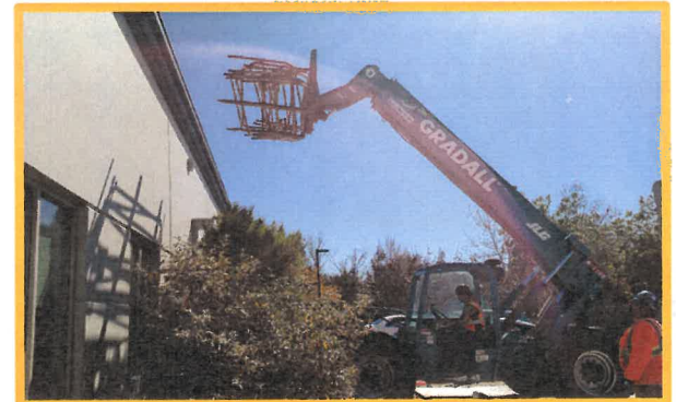
Moving Materials to Roof
