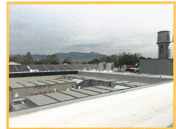
Lab Building Roof – HVAC and Solar Panels
