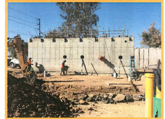
Wet Well Construction
