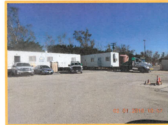
Contractor Mobilization at RP-1 Headworks
