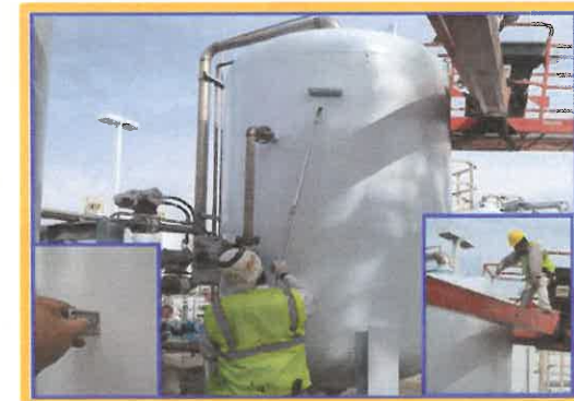
Finish Coat to Process Tanks
