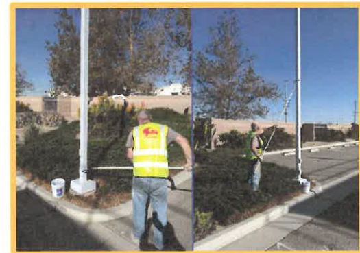
Finish Coat to Light Poles
